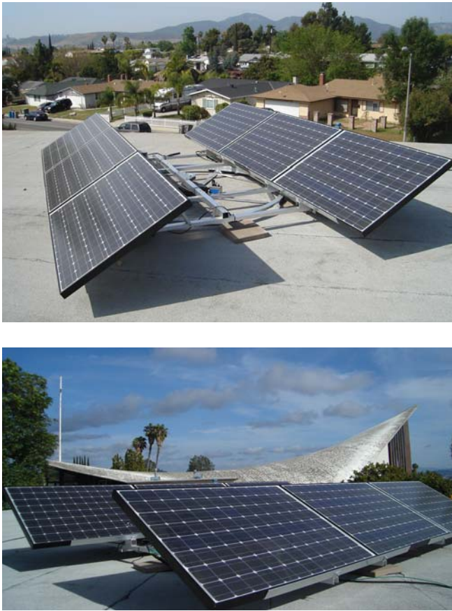
Figure 5: Two views of a 1.2 kW (peak DC) JXC SunTrack Carousel mounted on a church rooftop in San Diego CA.
